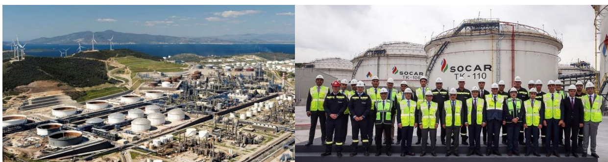
Figure 12: SOCAR STAR Refinery (Turkey).
