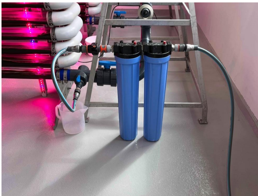
Figure 5. This image shows a dual-stage water filtration system installed in a pilot facility for cultivation of microalgae in tubular photobioreactors. The system features two blue filter housings (1 and 0.3 micron) connected to input and output hoses, ensuring efficient water purification.
